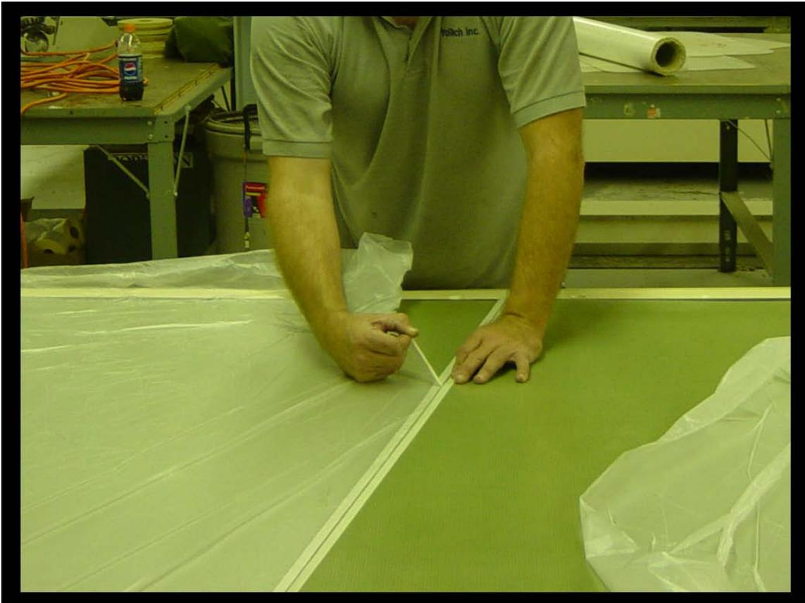
11. Bond the joint together by applying downward pressure with a roller or the face of a hammer, be thorough and go over the entire joint at least twice.
